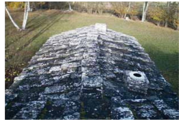
Fig 5.1 Flistak Gotland
